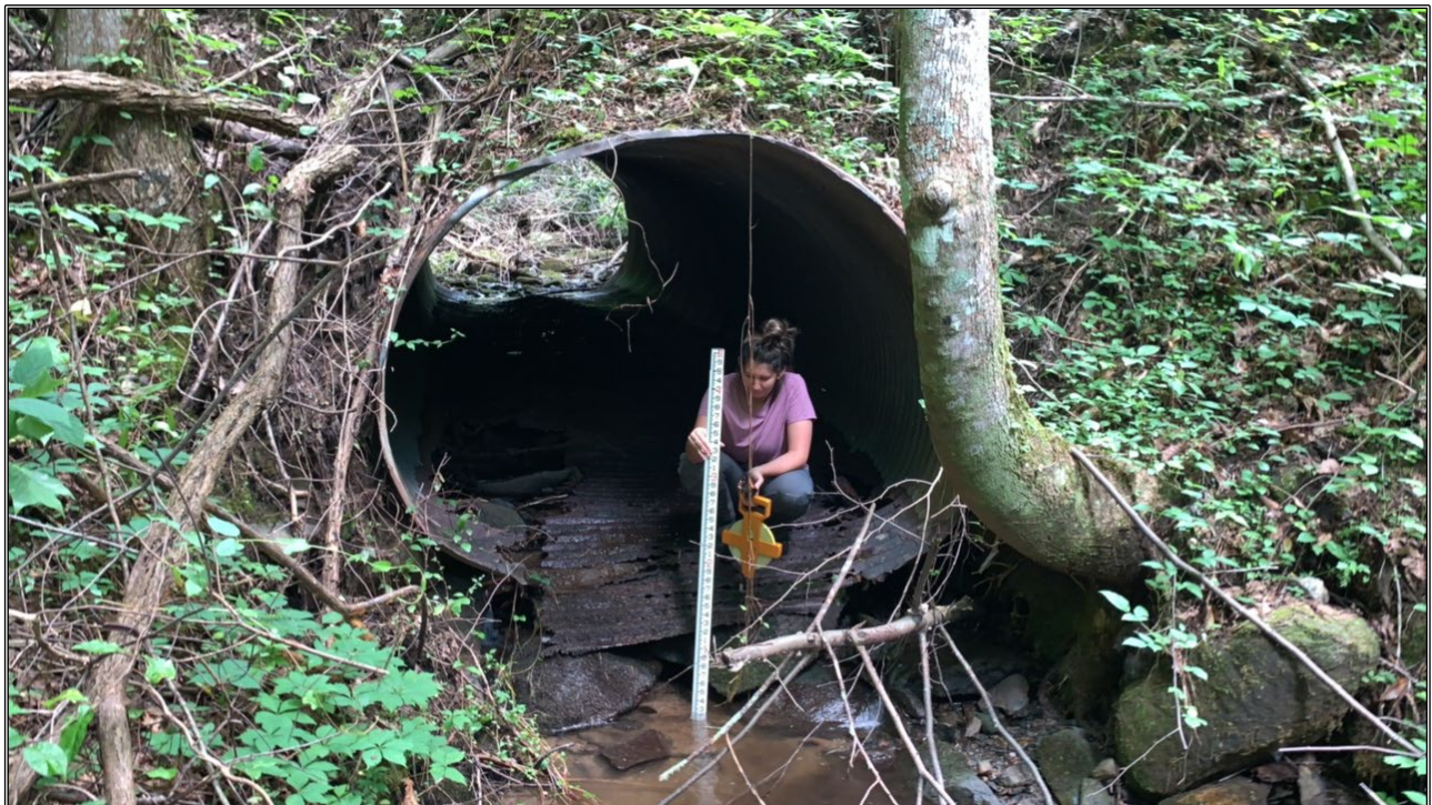
AOP candidate on Milma Branch. This culvert is a complete barrier to aquatic organism passage.
